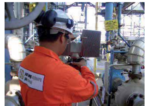
PD Engineers uses the Laser Scanner LS from FARO Technologies
